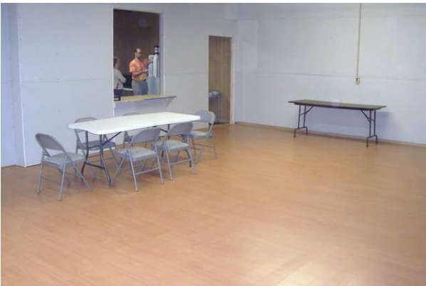
Drywall added over frame, hole cut for service
