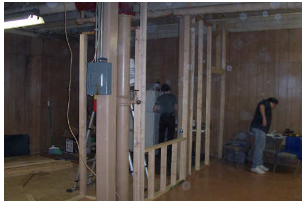
Framing the classroom wall
