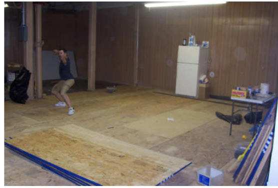
Adding the subfloor for the classroom
