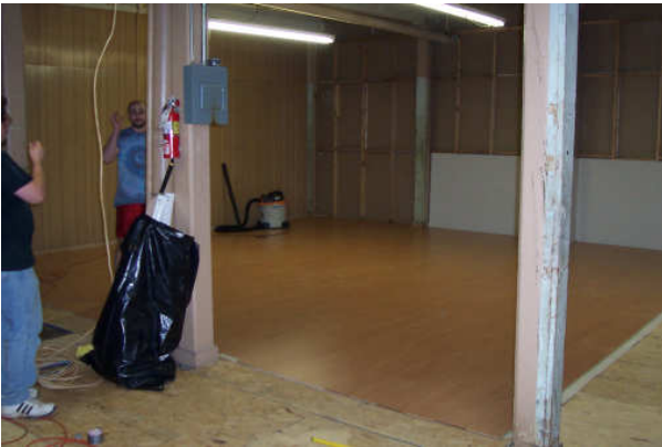
Adding the laminate flooring over subfloor
